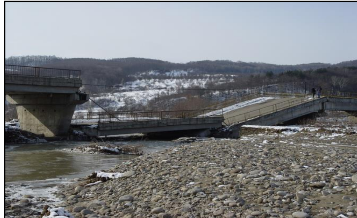
Effects of the flood in May, 2005 - breaking a bridge over Bâsca Chiojdului River, Buzau R.B.
